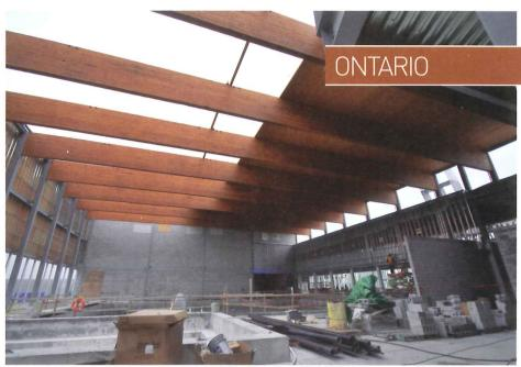
The incorporation of a CLT roof system is thought to be the first commercial use of CLT in Ontario. Cross-laminated timber panels (CLT) and re-used glulam roof beams were used to construct the roof system over the new pool area. The project design team made the decision
