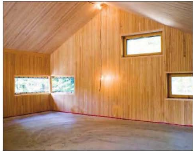
The Austria House (Whistler, B.C.) features the first Canadian application of cross-laminated timber (CLT) panels for roof and floor structure and diagonally dowelled solid wood panels for the wall structure.
