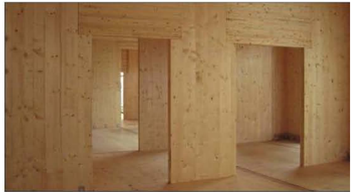
CLT panels can be assembled in platform-frame fashion, like concrete slabs suspended between load-bearing walls.
